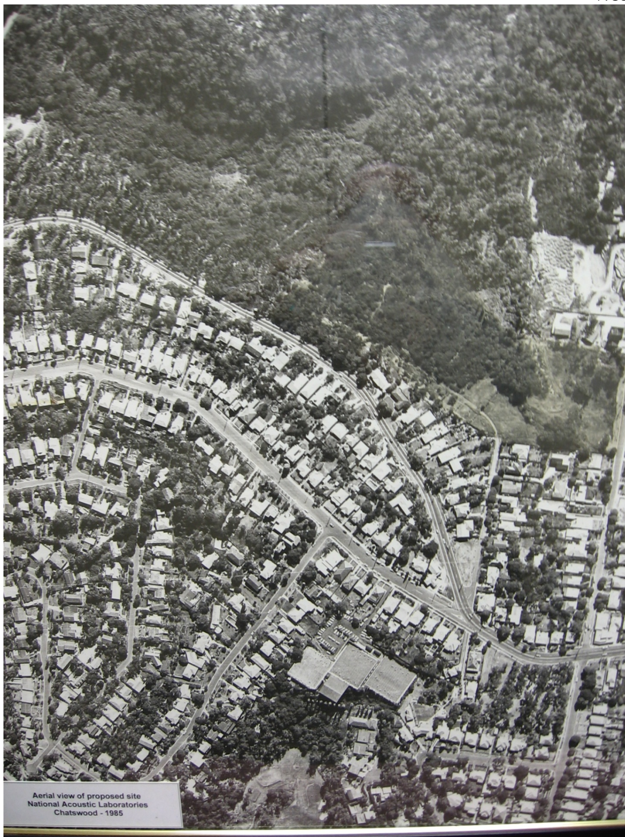
Figure 7 - 1985 Aerial photograph of the site showing site conditions just before construction of the National Acoustic Laboratory and Ultrasonics Institute commenced
